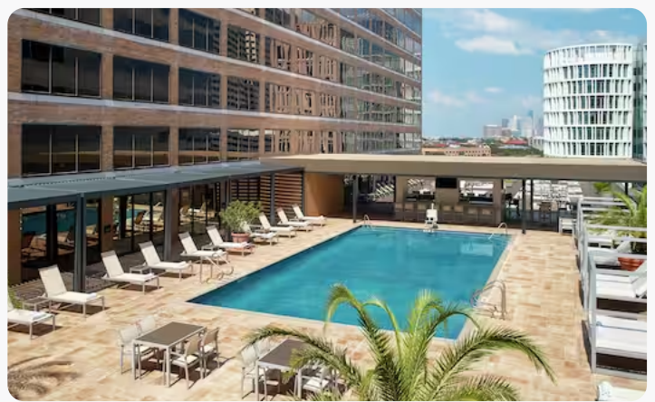
Swimming Pool Facing
